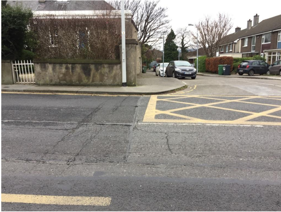
Figure 2.23: Example of poor road conditions on Monkstown Road at entrance of Montpellier Manor
