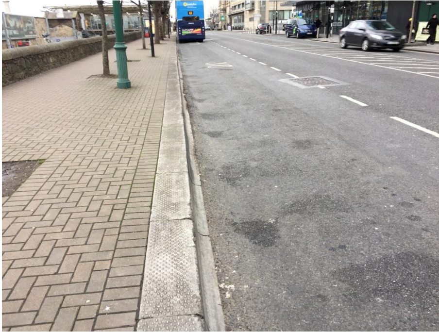
Figure 2.36: Road in poor condition at the bus stop on Crofton Road
