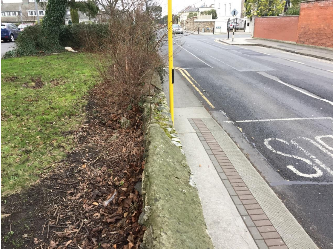
Figure 2.30: Retaining Wall at Montpellier Parade
