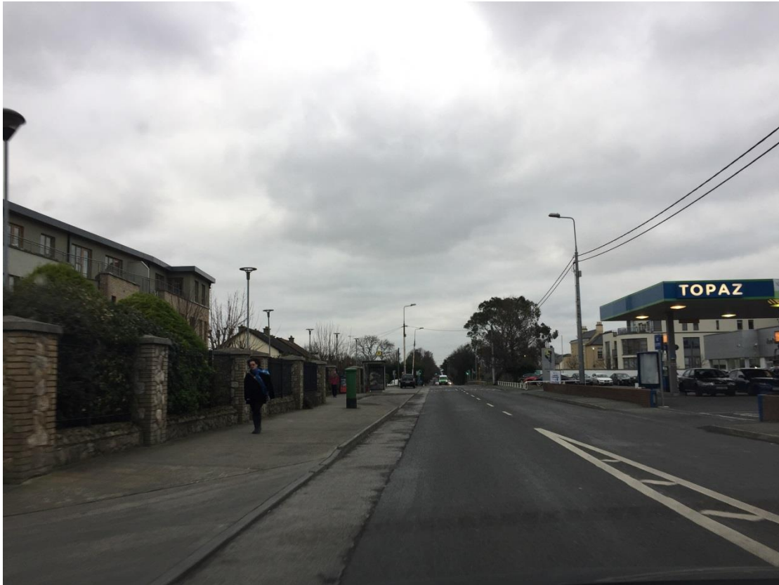
Figure 2.9 Example of poor road condition along Rochestown Avenue
