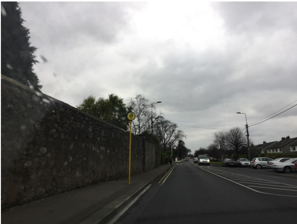
Figure 2.11: Example of footpath with reduced width on Rochestown Avenue opposite Killiney Shopping Centre
