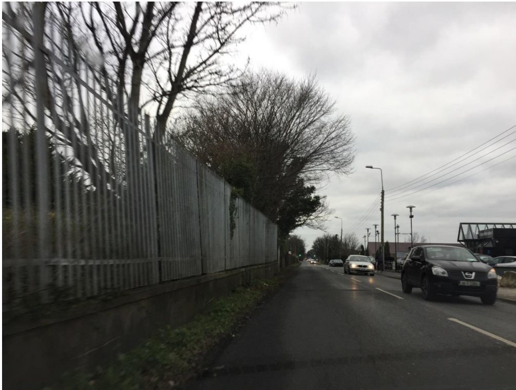
Figure 2.13: Lack of footpath facilities on Rochestown Avenue
