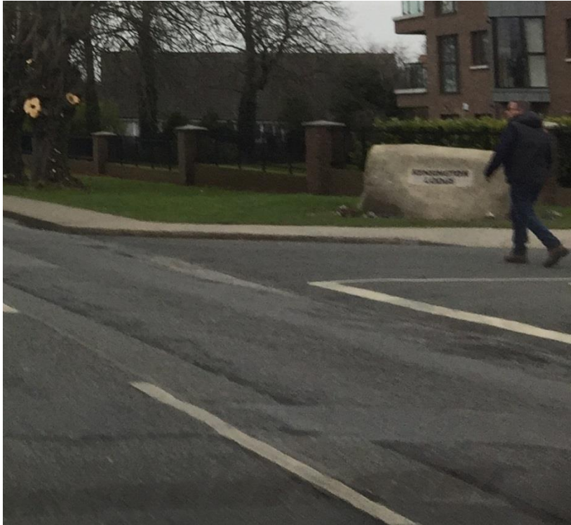
Figure 2.15: Lack of tactile paving at the crossing point at entrance to Kensington Manor
