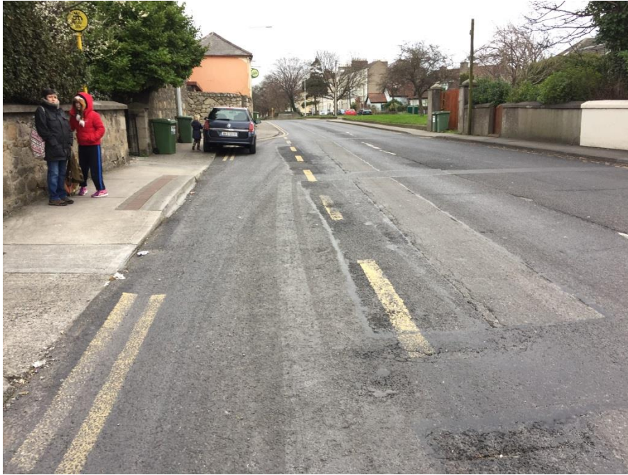
Figure 2.22: Example of poor road conditions at bus stop on Monkstown Road
