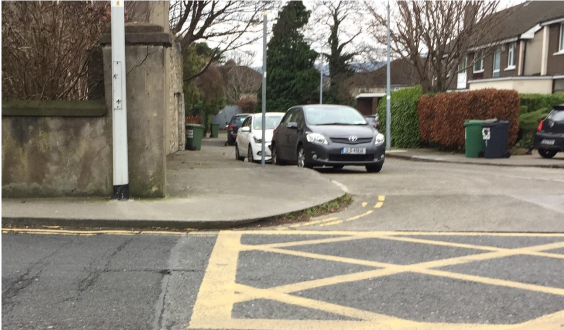
Figure 2.29: Entrance to Montpellier Manor illustrating lack of tactile paving
