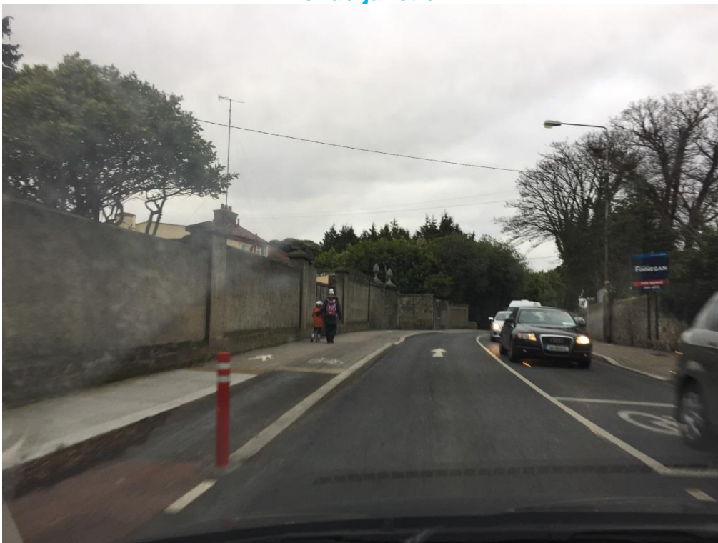
Figure 2.8: Shared surface footpath Stradbroom Road
