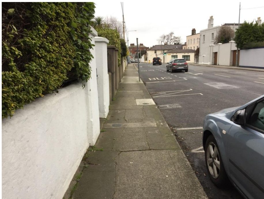
Figure 2.38: Footpath in poor condition Newtown Avenue
