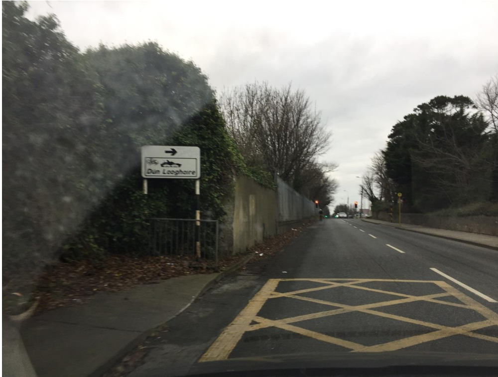
Figure 2.12: End of footpath opposite Somerton residential estate
