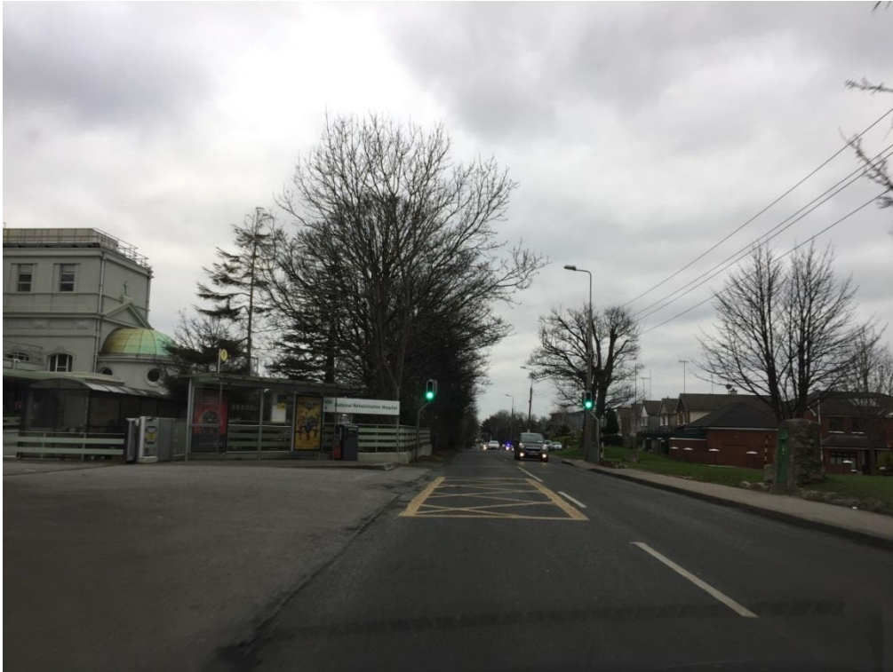
Figure 2.10: Dilapidated road condition at entrance to National rehab Centre
