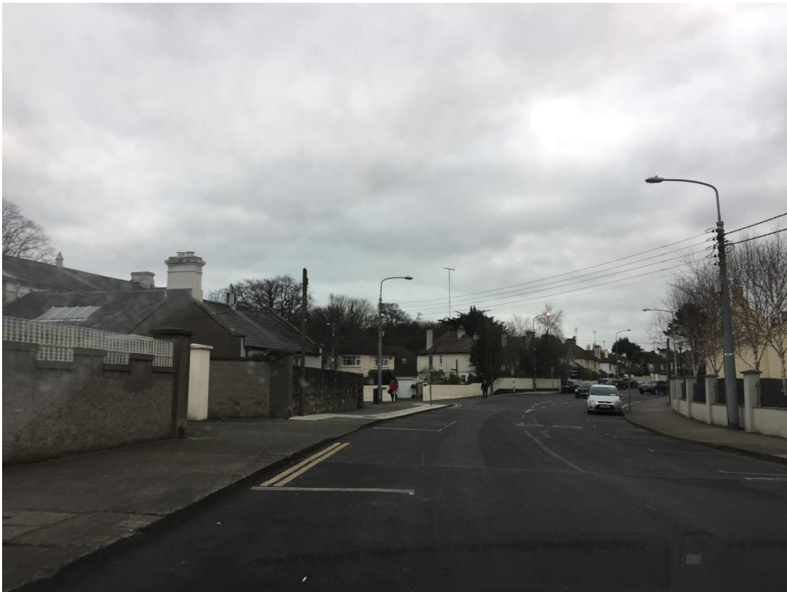
Figure 2.20: Example of lack of cycle facilities on Carrickbrennan Road
