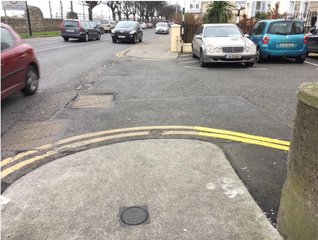
Figure 2.39: Lack of tactile paving at Crofton Road/Stable Lane junction
