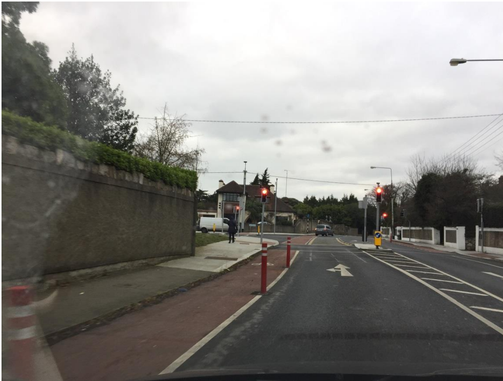
Figure 2.7: Cycle facilities on approach to Stradbroom road/Newtownpark Avenue junction
