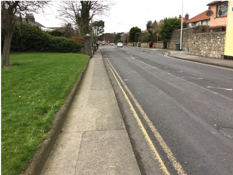
Figure 2.27: Section of dilapidated footpath Monkstown Road
