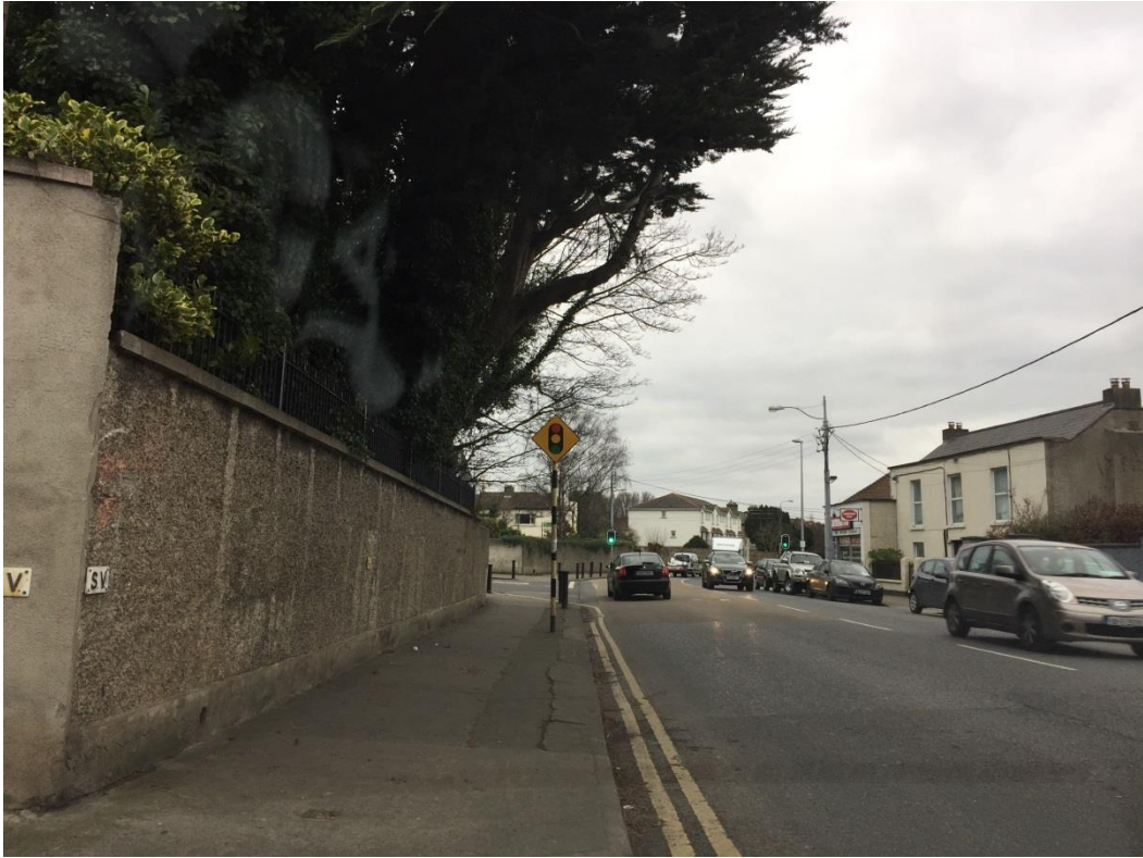
Figure 2.28: Section of dilapidated footpath on Mounttown Road Lower
