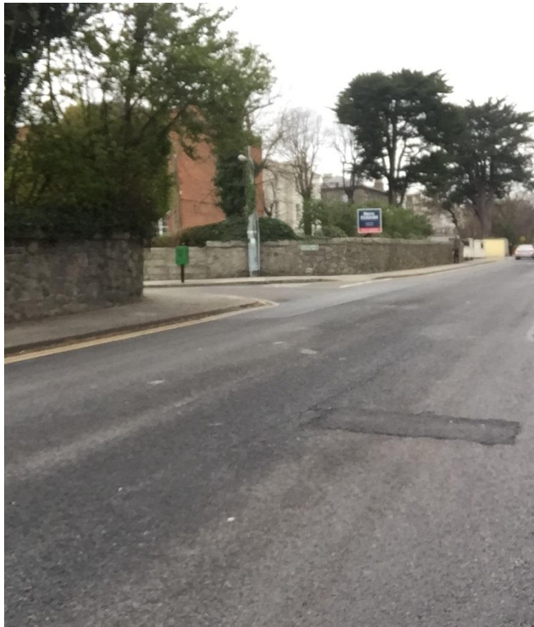
Figure 2.24: Road condition looking East-West on Monkstown road
