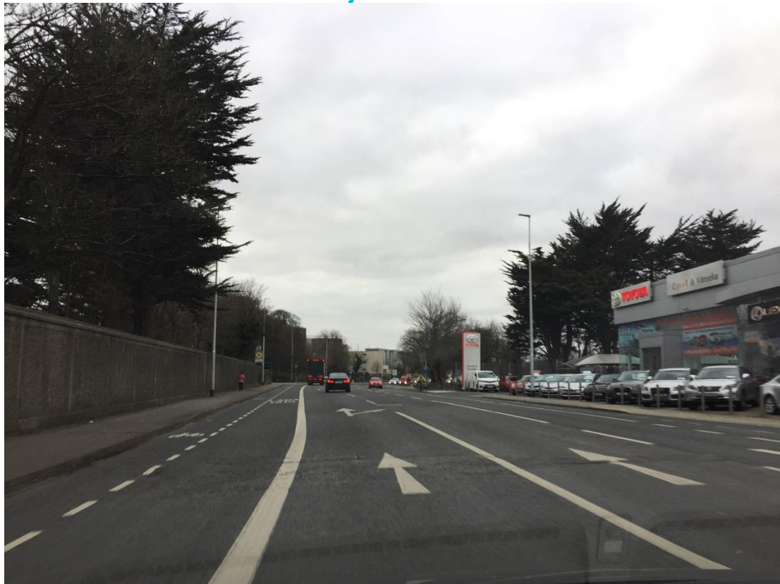
Figure 3.3: Example of the lack of thermoplastic material in cycle track on Rock Road
