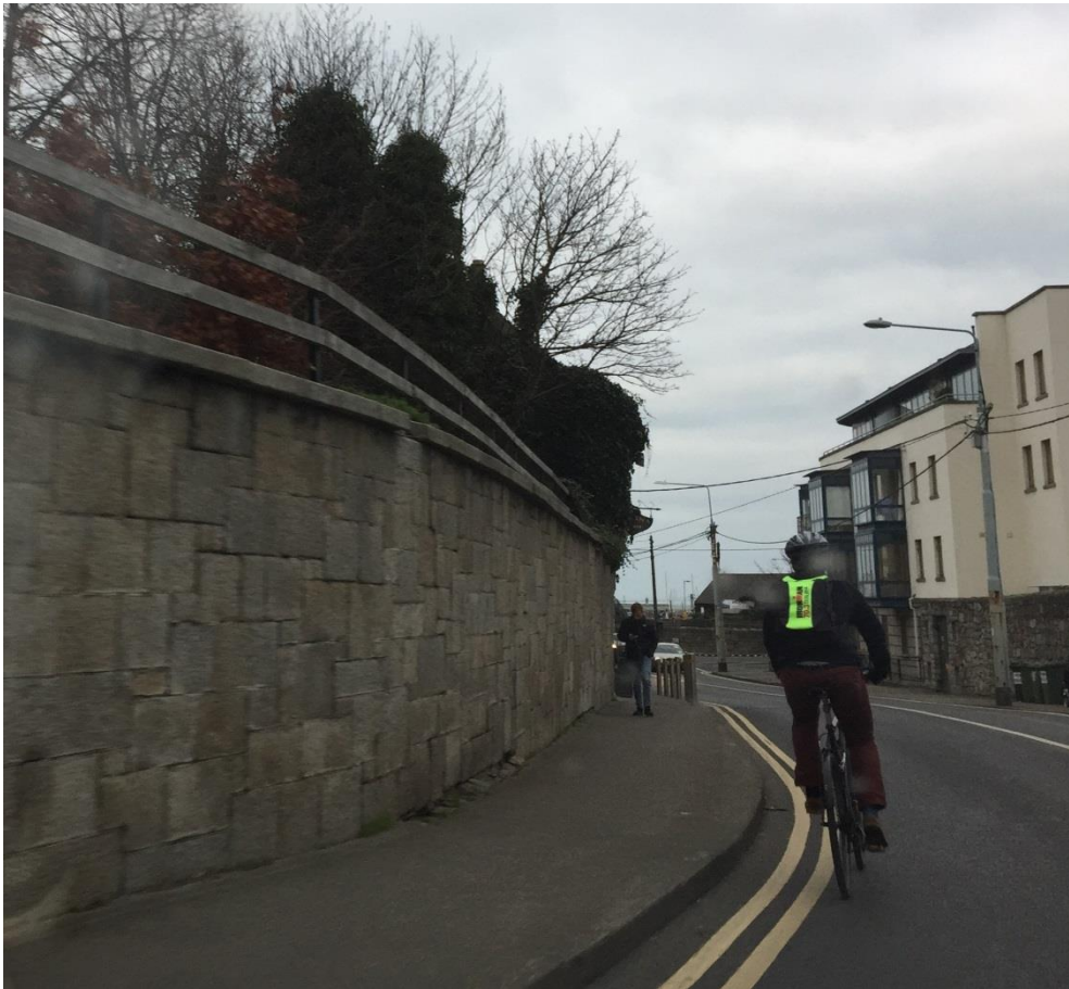
Figure 2.40: Retaining Wall Old Dunleary Road
