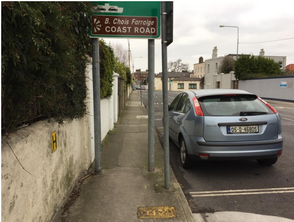
Figure 2.37: Traffic sign upright causing obstruction in footpath Newtown Avenue
