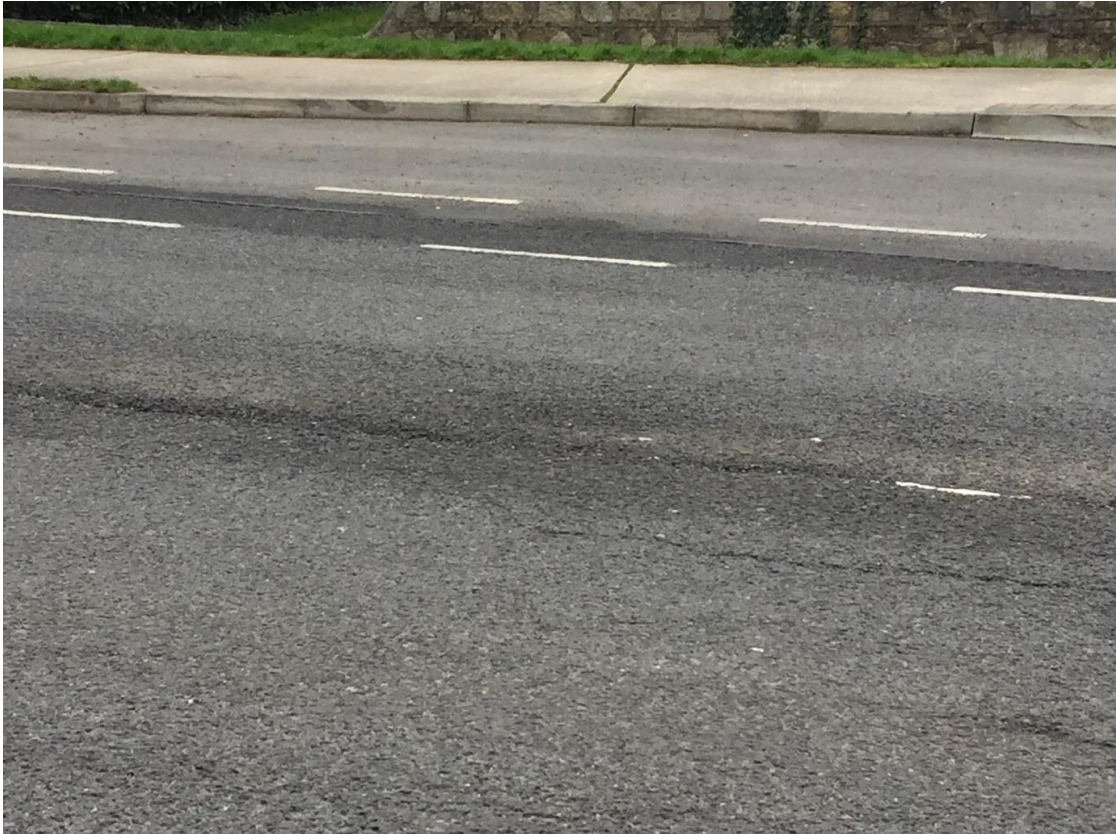
Figure 2.25: Poor road condition Mounttown Road Upper
